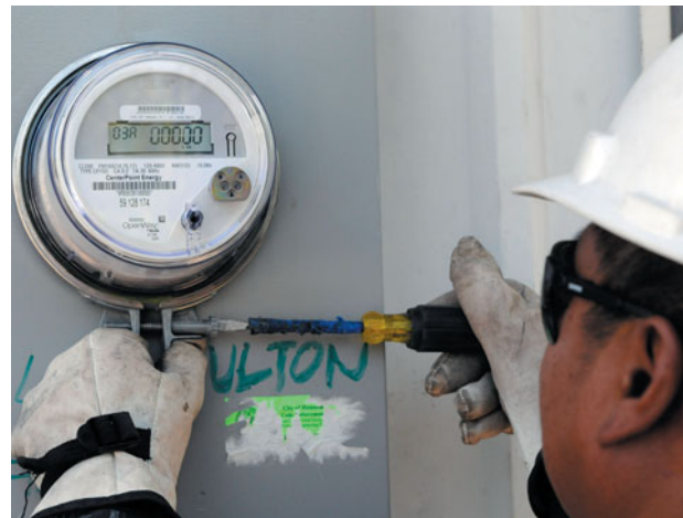
A smart meter being installed
