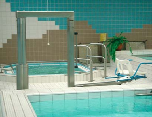
Fig. 2.6. Many hydrotherapy units are equipped with instrumentation for controlled lowering of patients with poor mobility to the pool
