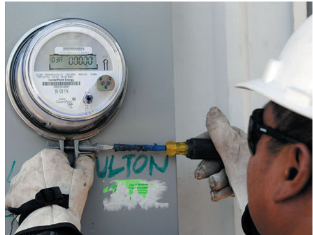
A smart meter being installed
