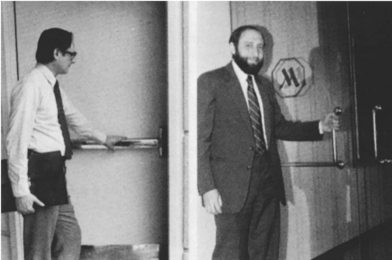
Figure 17.5 Affordances of Doors. Door hardware can signal whether to push or pull without signs. The flat horizontal bar of A (above left) affords no operations except pushing: it is excellent hardware for a door that must be pushed to be opened. The door in B (above right) has a different kind of bar on each side, one relatively small and vertical to signify a pull, the other relatively large and horizontal to signify a push. Both bars support the affordance of grasping: size and position specify whether the grasp is used to push or pull—though ambiguously.
