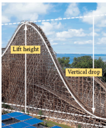
This is the first hill of the Mean Streak at Cedar Point.
